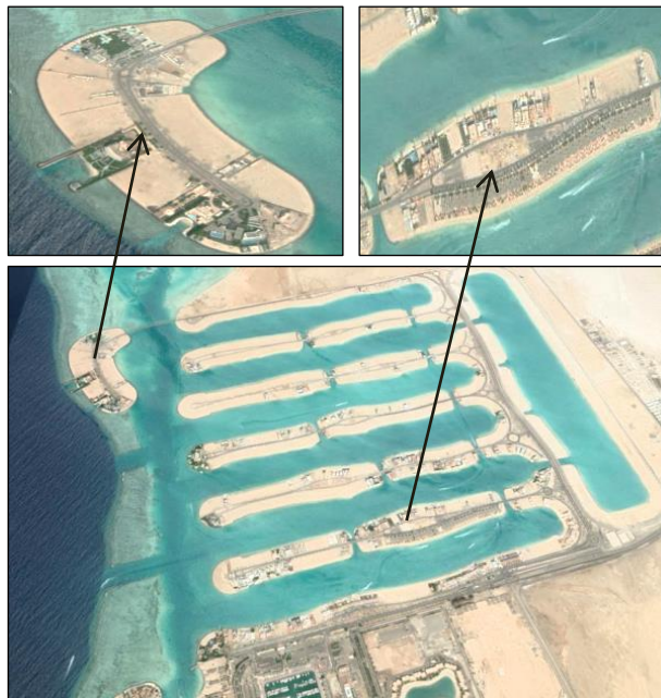
Source: The researcher's work based on satellite images Figure (5) Engineering Planning of Durrat Al-Arous Project
